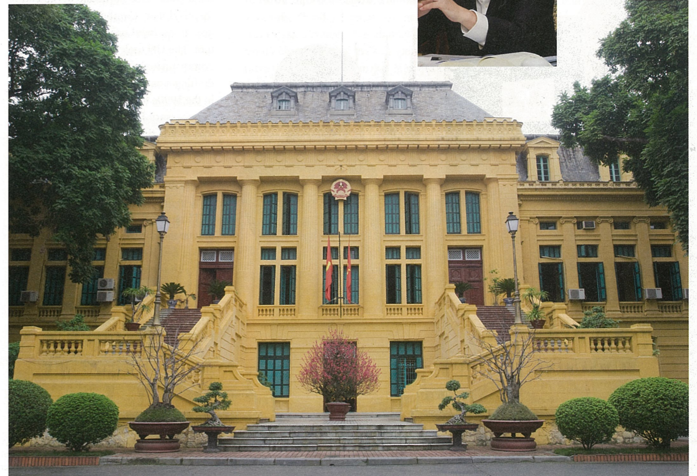
The French colonial architecture is defining characteristic of the Supreme People's Court of Vietnam.
